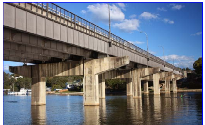
Figtree Bridge: Redundant concrete supports for the Lane Cove Valley Expressway
