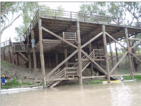
Bourke wharf, designed for times when the river was considerably higher
