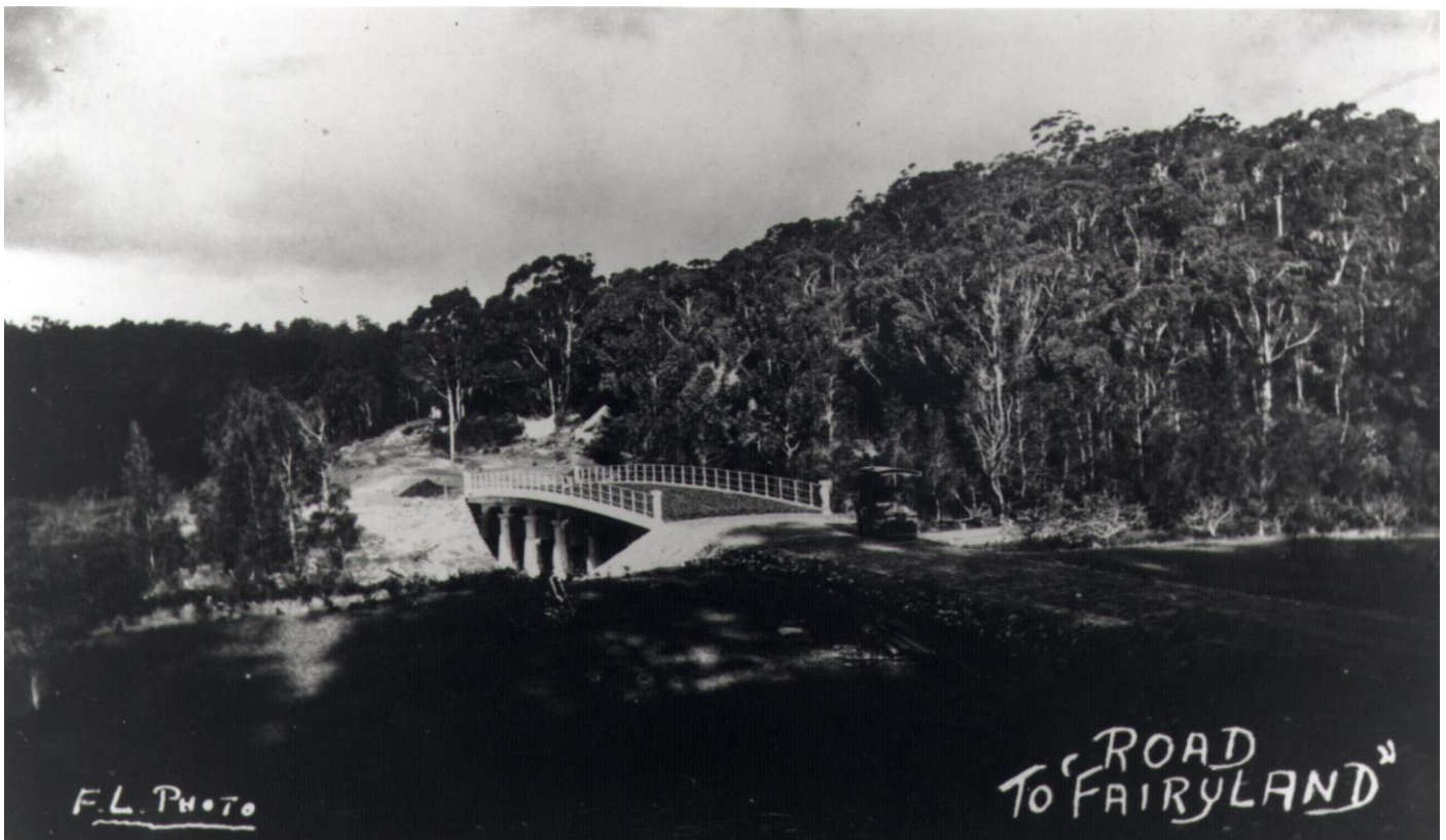
Above: Fullers Bridge nearing completion circa 1918 (Source – City of Ryde Library ref 5095778)
