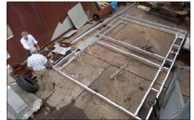
Jeremy Spear (rear) and Tom Sims from Sydney Marina Contracting check the aluminium frame which holds the two new downstream pontoons together.
