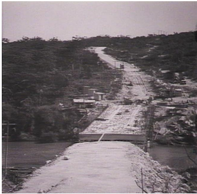
Above: Epping Bridge Construction – looking West towards Epping.
