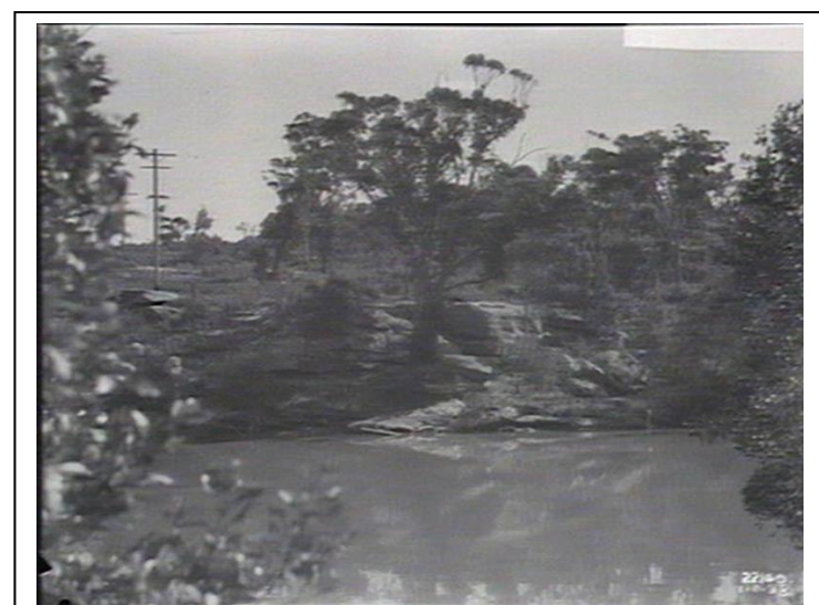
Above: Bridge Site September 1938 – looking from Timekeepers position to opposite bank and intended road alignment up the hill alongside the power pole. Source: Government Printing Office 32362. Copyright State Library of NSW. http://acms.sl.nsw.gov.au
