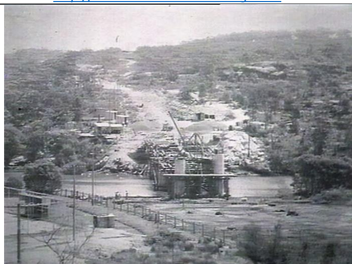
Above: Bridge under construction Feb 1939 - looking west across the Lane Cove River. Duck corner factory at left – LCRK car park at right.
