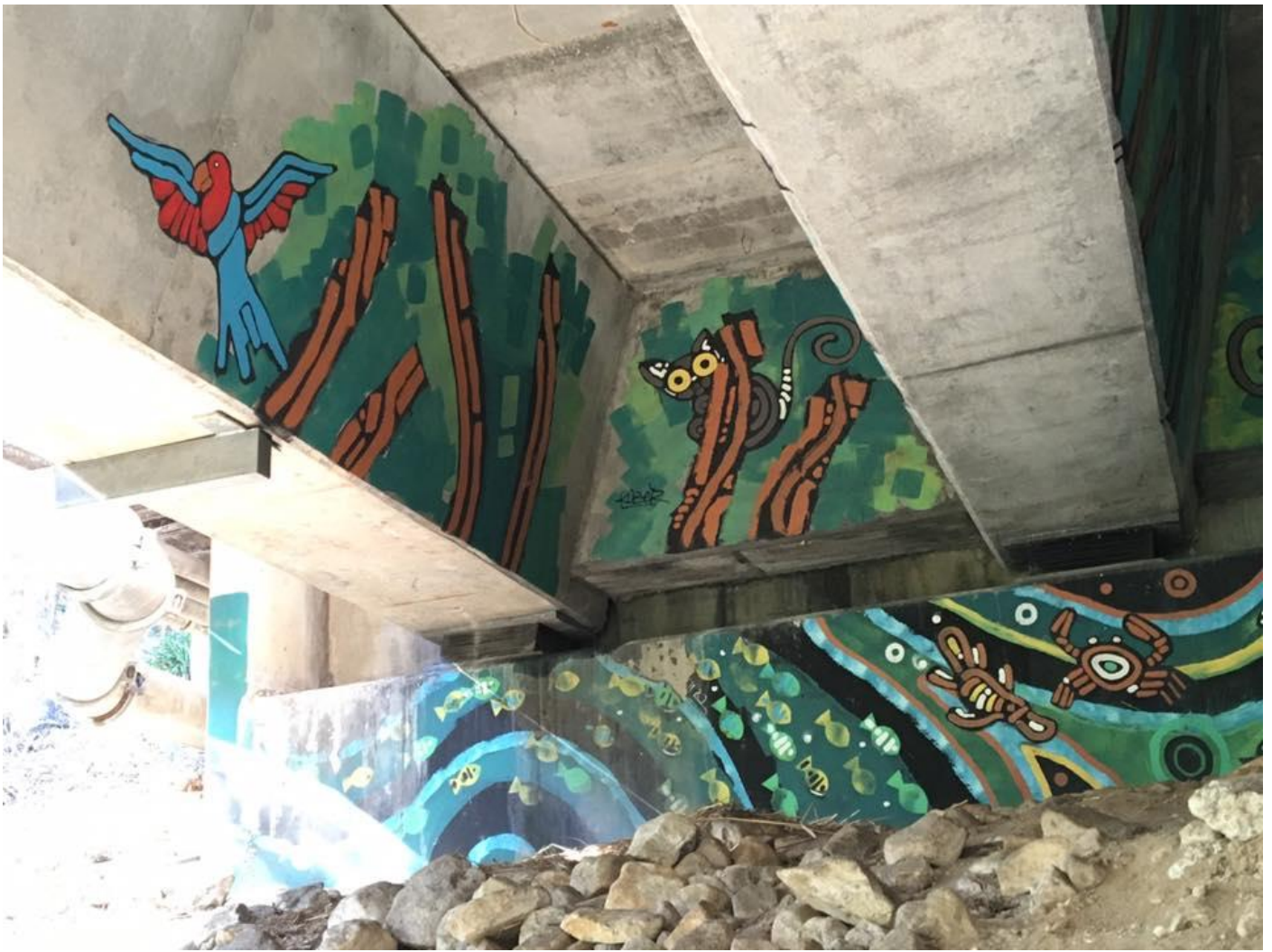
Above: The underside of Epping Bridge – decorated by someone with some flare, and some paint... Source: Image by member Maya Gibson
