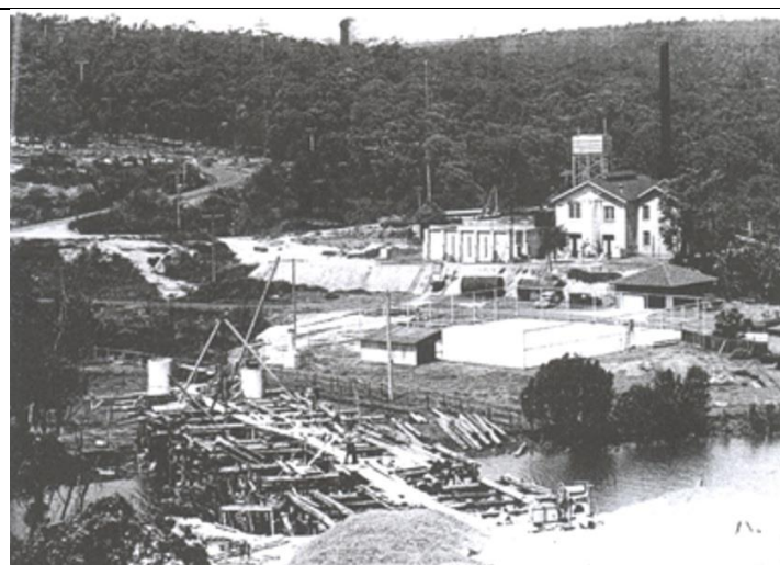
Above: Epping Bridge under construction Feb 1939– looking east across the river to Timekeepers Position. Factory at Duck Corner on the right with corn mill boiler house, coal bunker, garage and tennis courts.
